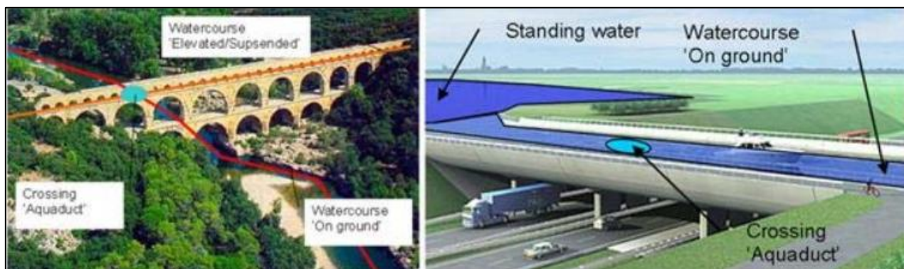
Figure 5 : Aqueduct with two watercourses crossing each other (source: www.lesstrainer.nl ) and aqueduct crossing a road (water still on ground level) - Extrait de la spécification Inspire illustrant la position par rapport au sol : « D2.8.1.8 Data Specification on Hydrography – Technical Guidelines »
